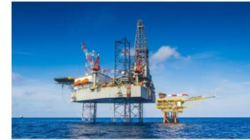
Gas and renewables have proven more resilient to the impacts of the pandemic than oil
